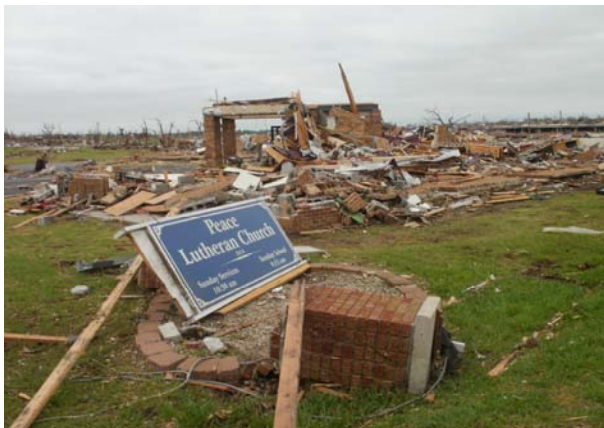
Tornado damage done to Peace Lutheran Church, Joplin, MO on May 22, 2011, destroyed the entire building.
